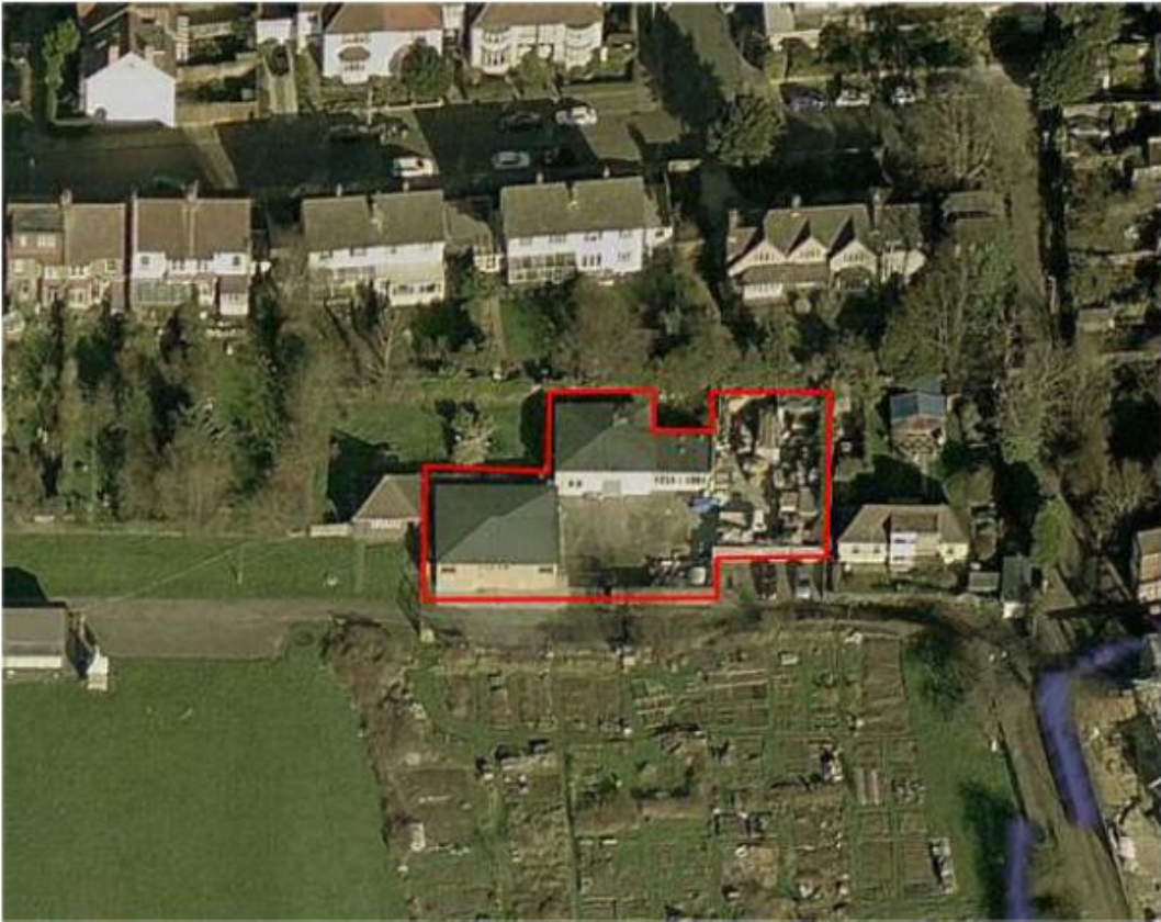
Aerial view of site
